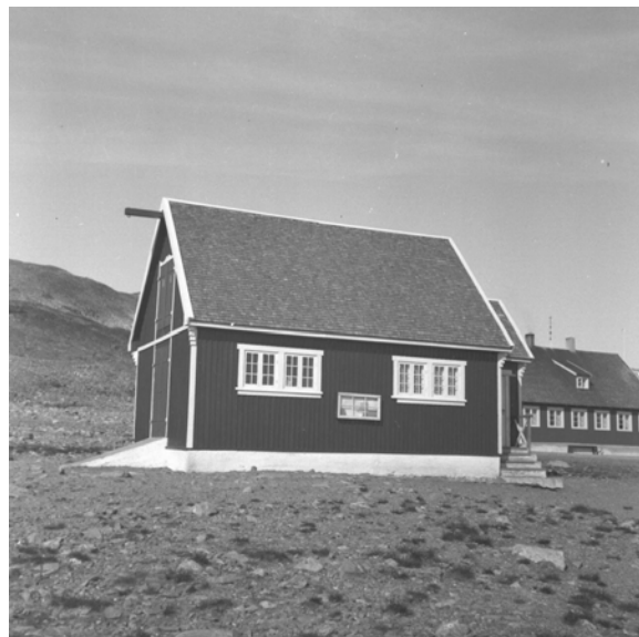
Figure 179 Noticeboard building with settlement manager Høegh's house in Scoresbysund (behind).
