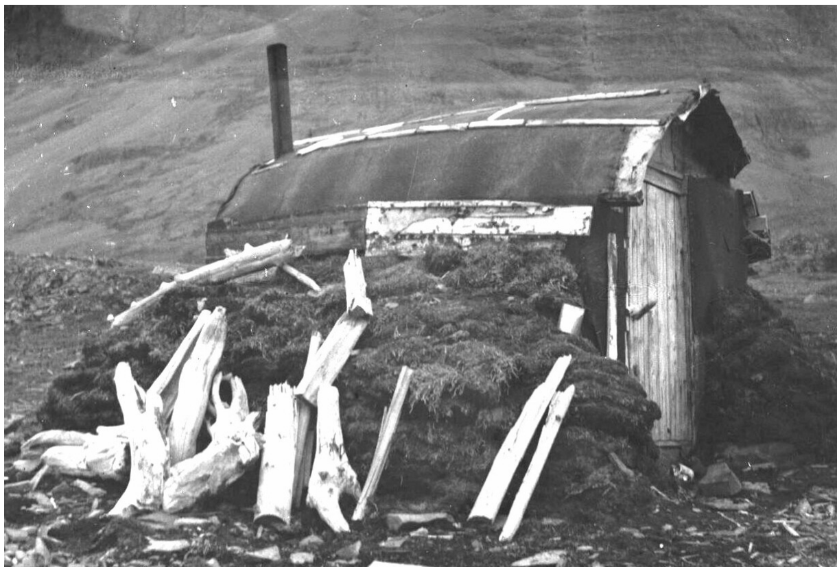
Figure 126 Hut at Kongeborg in Kong Oscars Fjord. The roof is an inverted boat outfitted with asphalt roofing felt, laths, etc. Driftwood is stacked up to dry against the earth protection
