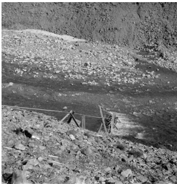
Figure 184 Water supply from river
