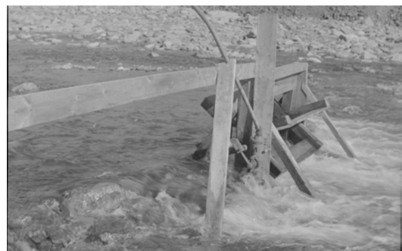
Figure 185 Water supply pump
