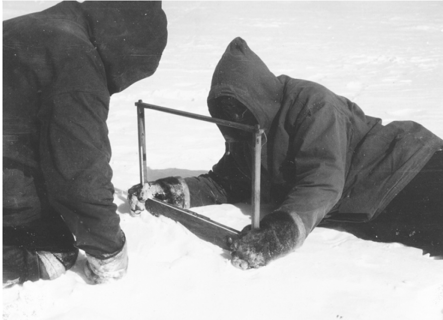
The 'Jakobs' baton' built by Sigurdsson to measure the sun's height after the loss of the theodolite. The ice sheet, May or June, 1913 (Photo: Arktisk Institut)
